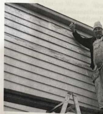
Geoff Hardy, Project Supervisor completed the west wall replacement well done by the committee.
