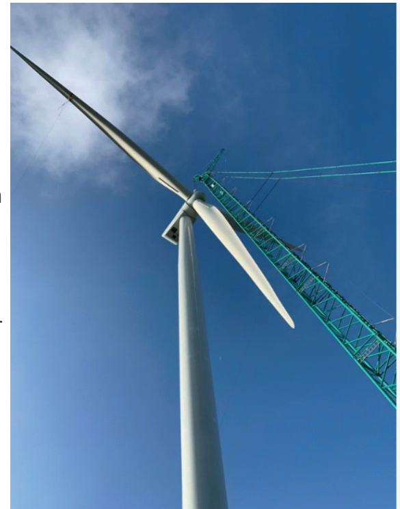
Image – Installation of Turbine 15 at MSWF
